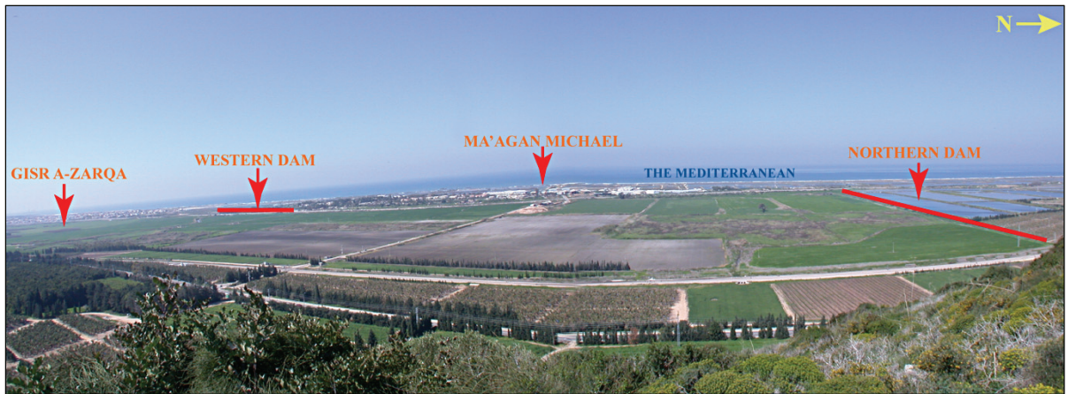
Fig. 2: The Tananim-reservoir area, looking west (photo and graphics – Y. Dray)
