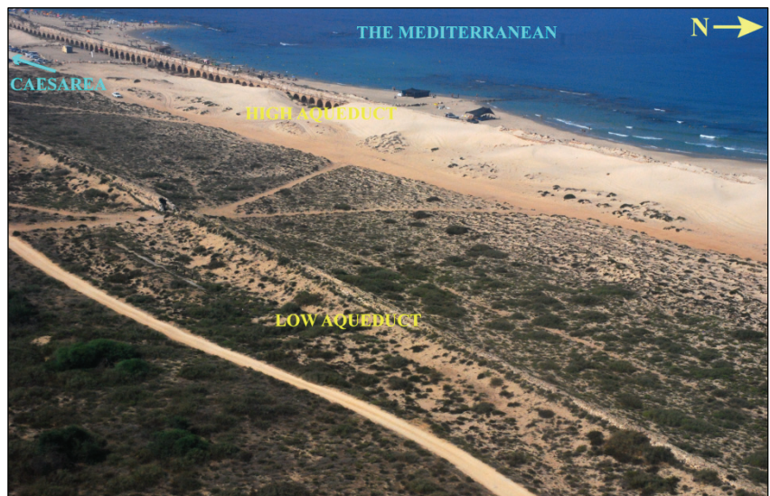
Fig. 9: ‘High level aqueduct’ and ‘low level aqueduct’ on their way to Caesarea (photo – A. Izdarechet; graphics – Y. Dray).
