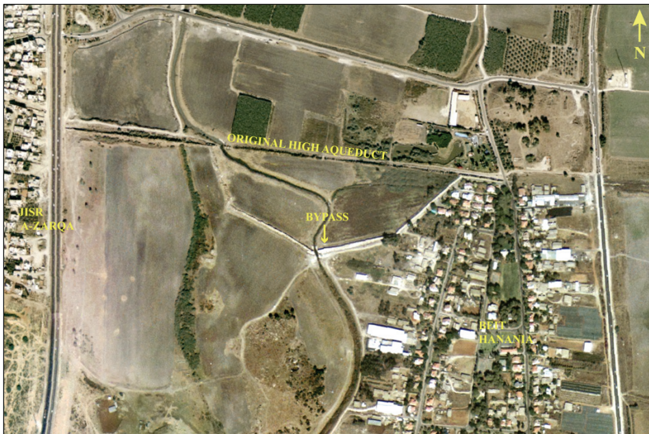
Fig. 12: The ‘high level aqueduct’ bypass (aerial photo – Ofek, courtesy of Carmel Drainage Authority; graphics – Y. Dray).
