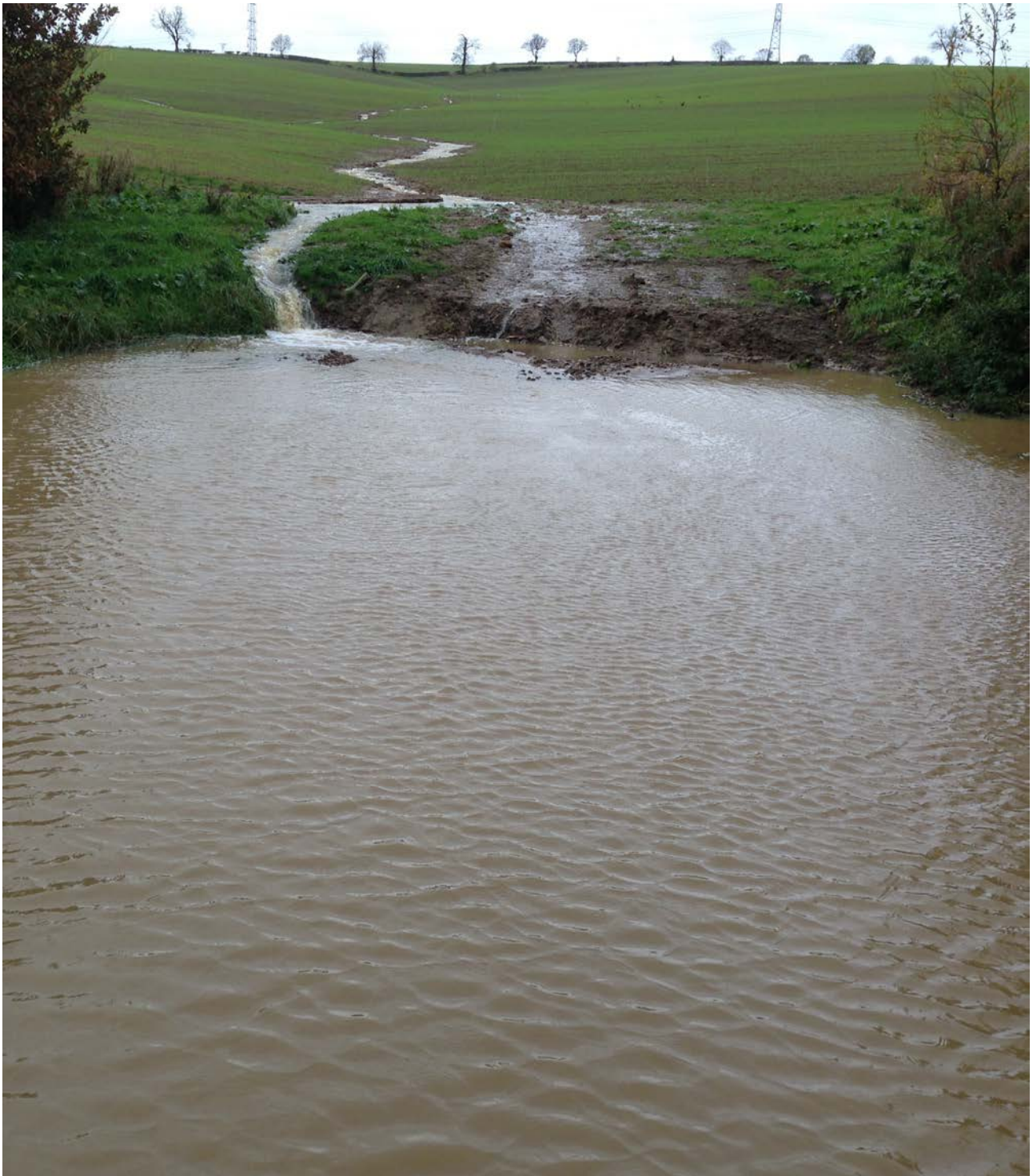
Figure 53. Field drain interception ponds. The picture shows a pond intercepting a field drain that previously discharged directly into the Eye Brook (behind photographer). This drain collects water from a field which represents about 5% of the arable area in Eye Brook project area. Note that there was overland flow and gulying along the line of field drain because the drain was too small to take the flows occurring at the time of the photograph (January 2013). This field drain was replaced with a larger diameter pipe in autumn 2014.
