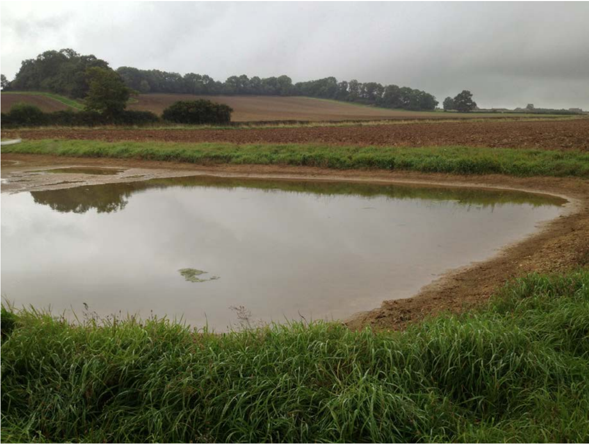
Figure 54. Flood storage basins. This flood storage basin detains water temporarily from the ditch draining the arable area behind the site, including the land upslope to the woodland.
