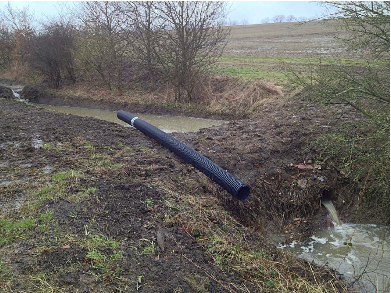
Figure 56. Large earth bunded ditch interceptor under construction.
