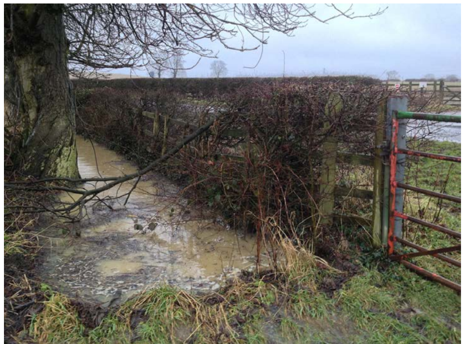
Figure 12b. Ditch draining into the Stonton Brook in wet weather in January 2013 transporting substantial quantities of sediment and associated pollutants to the stream network. Field drains are an essential part of the agricultural environment maintaining soils in a condition suitable for arable cropping.
