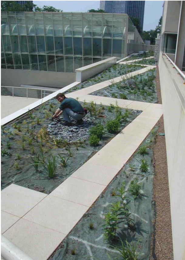
Peggy Notebaert Nature Museum Irrigation: Capillary fabric and Base level trickle irrigation
