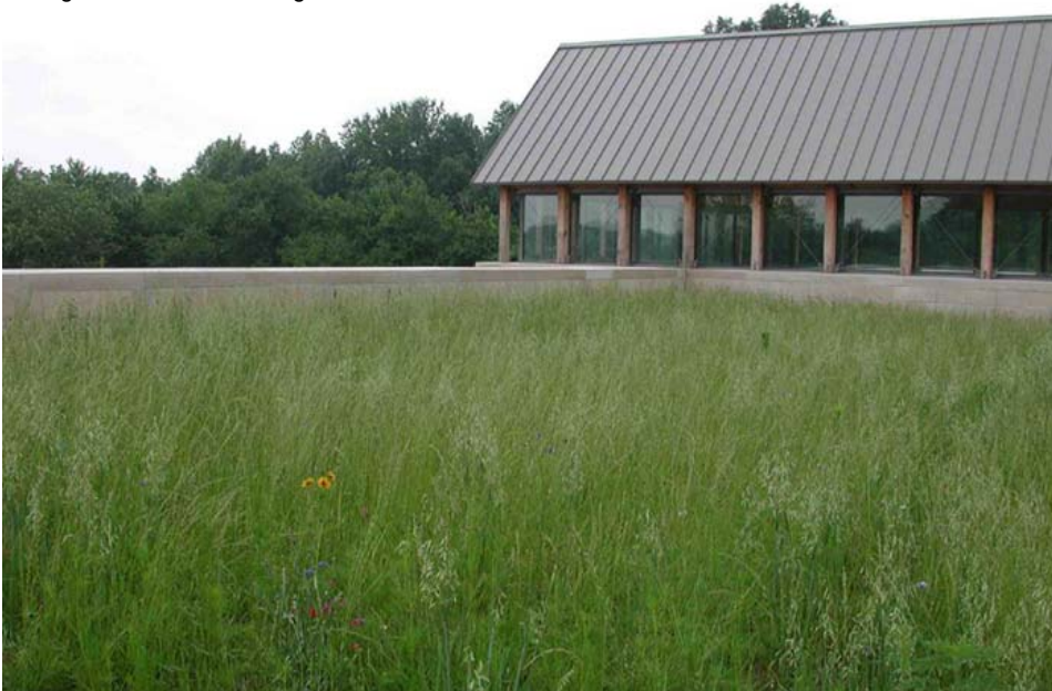
Oaklyn Branch Library Irrigation: Base trickle irrigation
